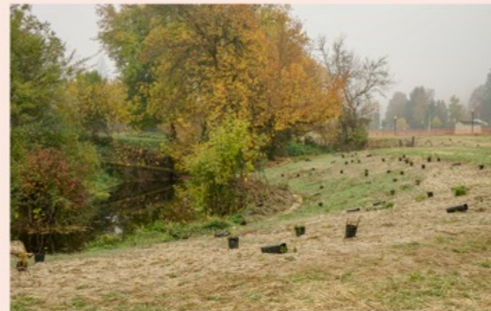
Stream restoration along South Scappoose Creek included pulling back incised banks to form shallower slopes and the addition of a large wood structure to create channel roughness. Photos show site with native vegetation prior to fall planting (left, top and bottom).
