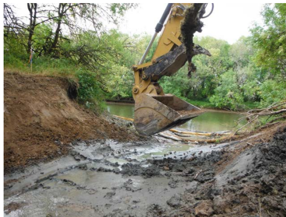
Photograph. Removing a culvert and berm to create a tidal channel outlet. Courtesy of T. Josephson.
