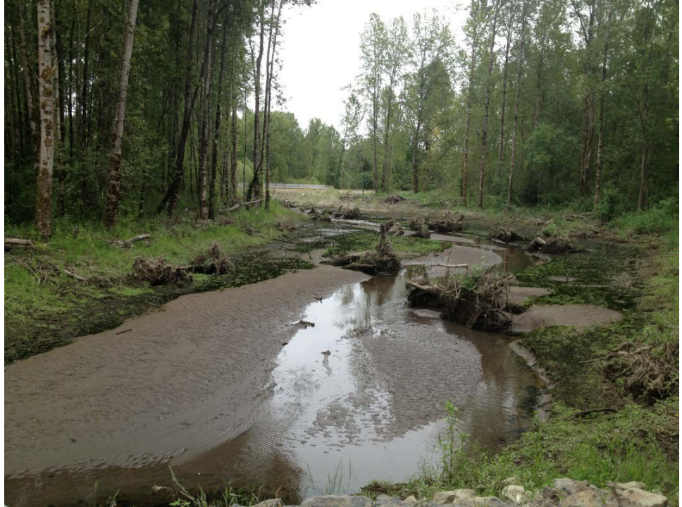
Excavated swale and stream channel
